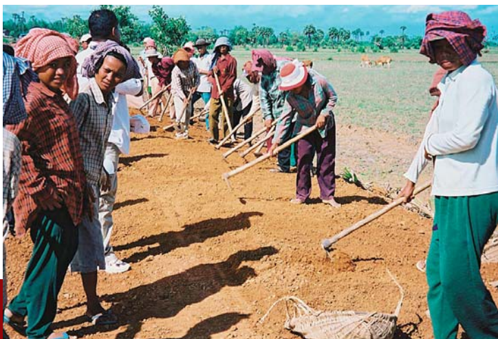
A joint effort: rural road construction
