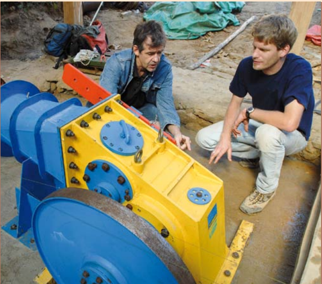
German engineers installing small hydro power plants contributing to rural electrification.
