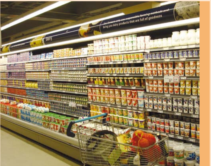
Pick’n Pay switched to energy-efficient refrigeration systems.
