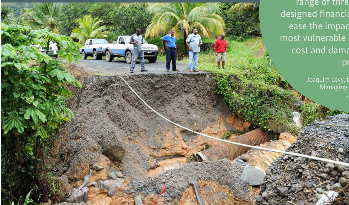
Losses after hurricane ‘Irma’ in 2017: damaged road in Dominica.
