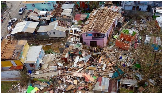
Storm damage on the Caribbean island of Dominica after Hurricane Maria in September 2017 © Ben Parker/IRIN via The New Humanitarian
