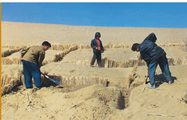
Dune stabilisation in Central Asia: communities stabilise sand dunes using desert flora and straw mats to protect their houses from sand encroachment
